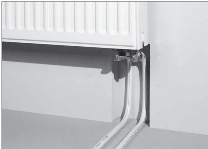
Radiator connection from the wall
