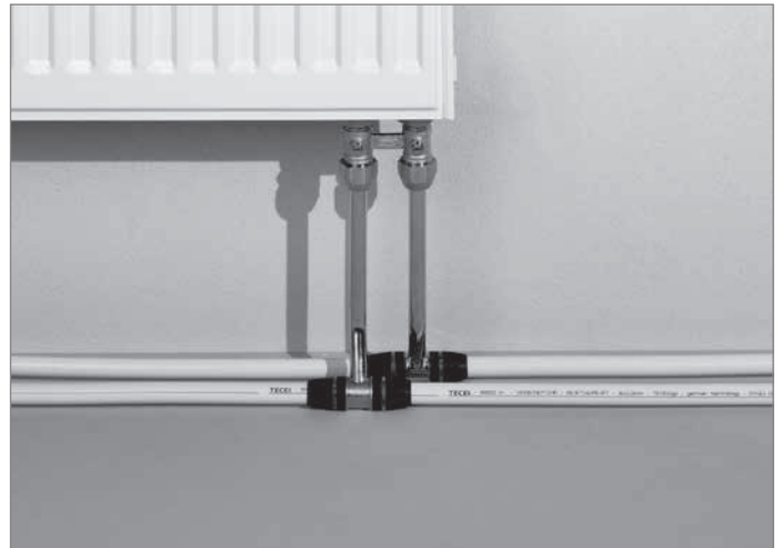
Radiator connection with radiator mounting tee
